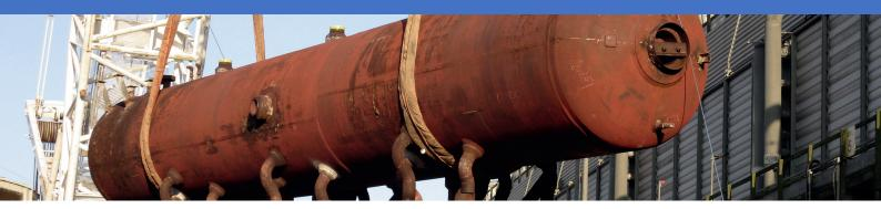
Unit Superheater Engineering (USE) undertook an extremely challenging repair and upgrade of two high pressure steam drums for the HRSG's at a CCGT plant in Runcorn, Cheshire.
