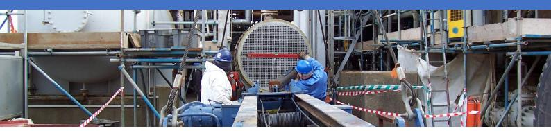
Unit Birwelco is a leading provider of bundle pulling services, be it for major shutdowns of 100 plus exchangers, spade-to-spade, or simple one-off pull and pushes.
